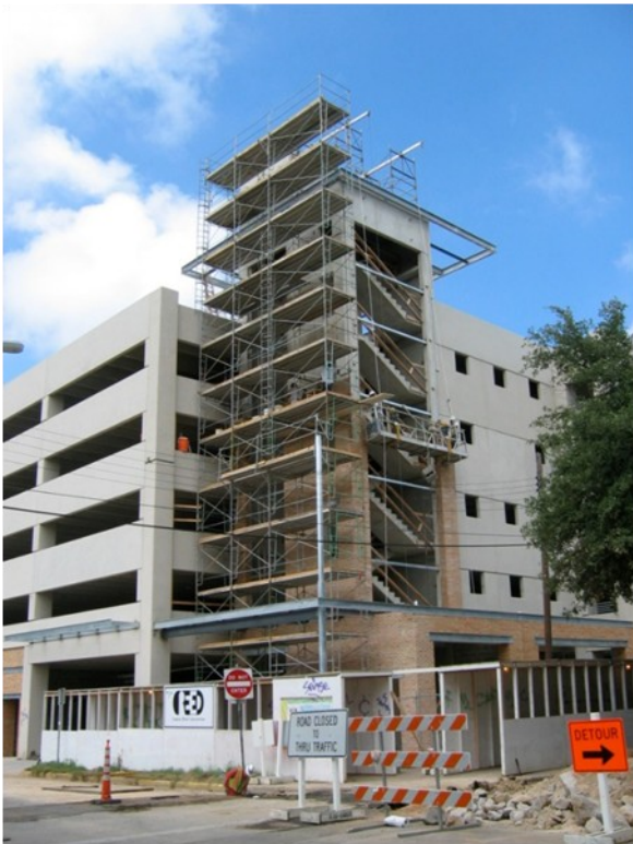
7/6/06 New parking garage going in across from the church
