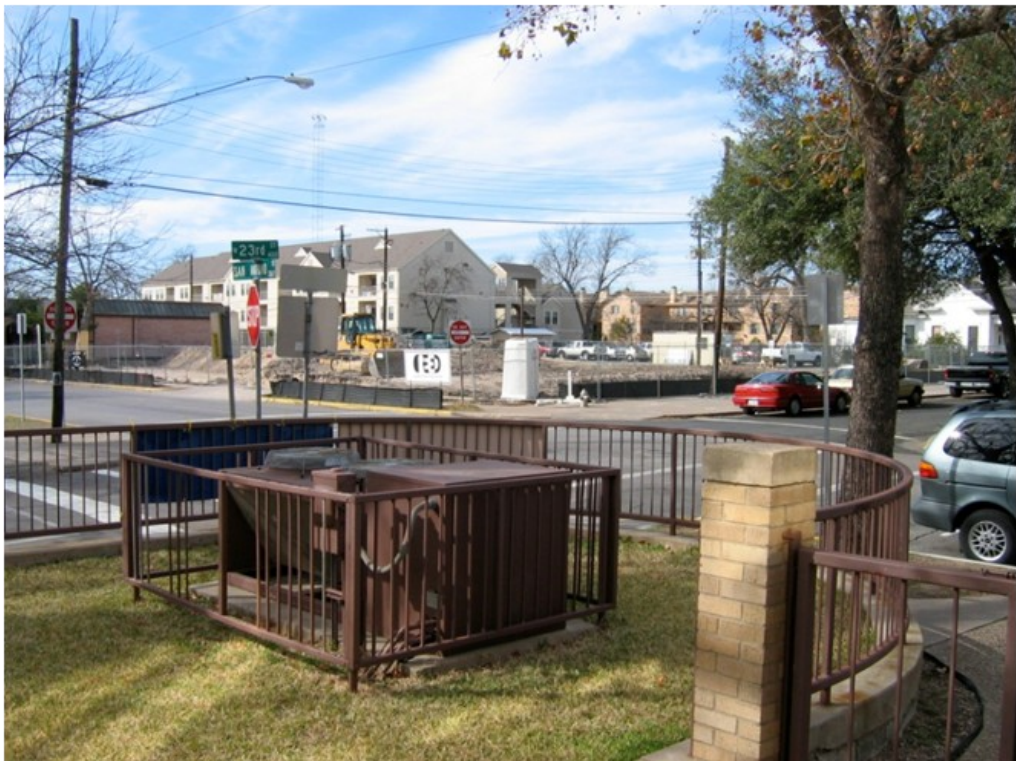
2/6/06 Construction on the parking garage diagonally across from the church
