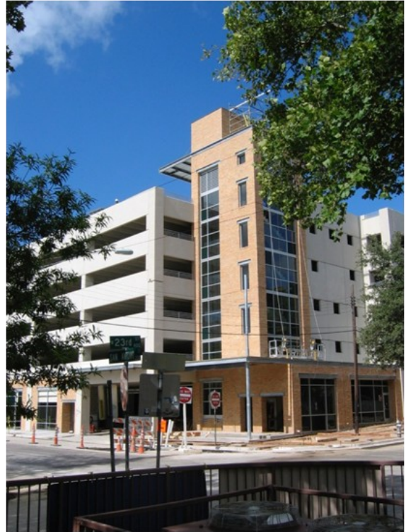
7/30/06 Further construction on the parking garage across from the church
