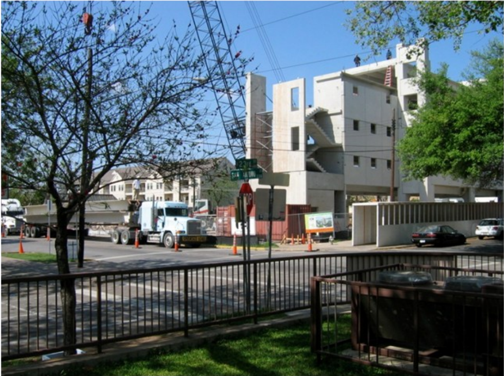
4/8/06 Parking garage across the street from the church undergoing construction
