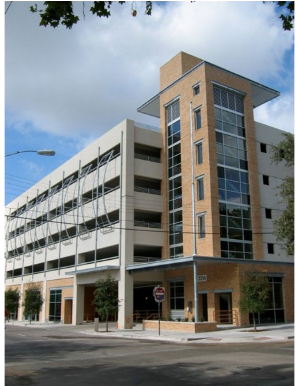
8/28/06 Finally— the completed parking garage across from the church
