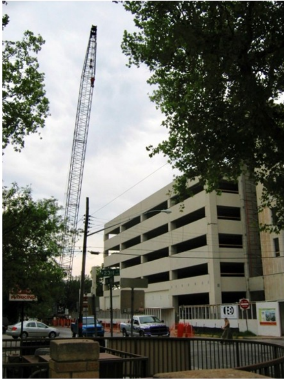
5/15/06 Construction on the new parking garage diagonally across the street from the church
